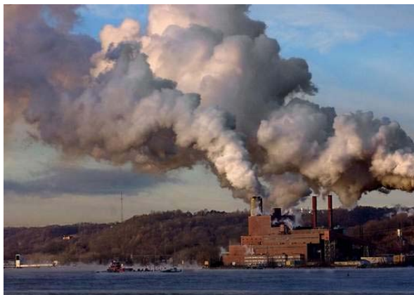
This 2004 photo shows the Danskammer electric power plant across the Hudson River, looking west from New Hamburg. The visible substance coming from the smokestacks is mostly steam, but emissions do include mercury. Mercury drops from the atmosphere can be converted to toxic forms such as methylmercury, which gets passed up the aquatic food chain to fish such as this brown trout. (File photo by Spencer Ainsley/Poughkeepsie Journal)
